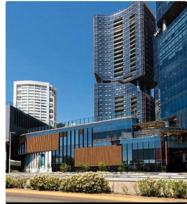
● Torre Mayor, Mexico City
